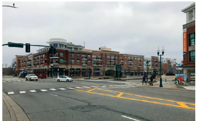
THE INTERSECTION PRIOR TO CONSTRUCTION
